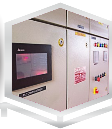
PLC EB/DG control panel
